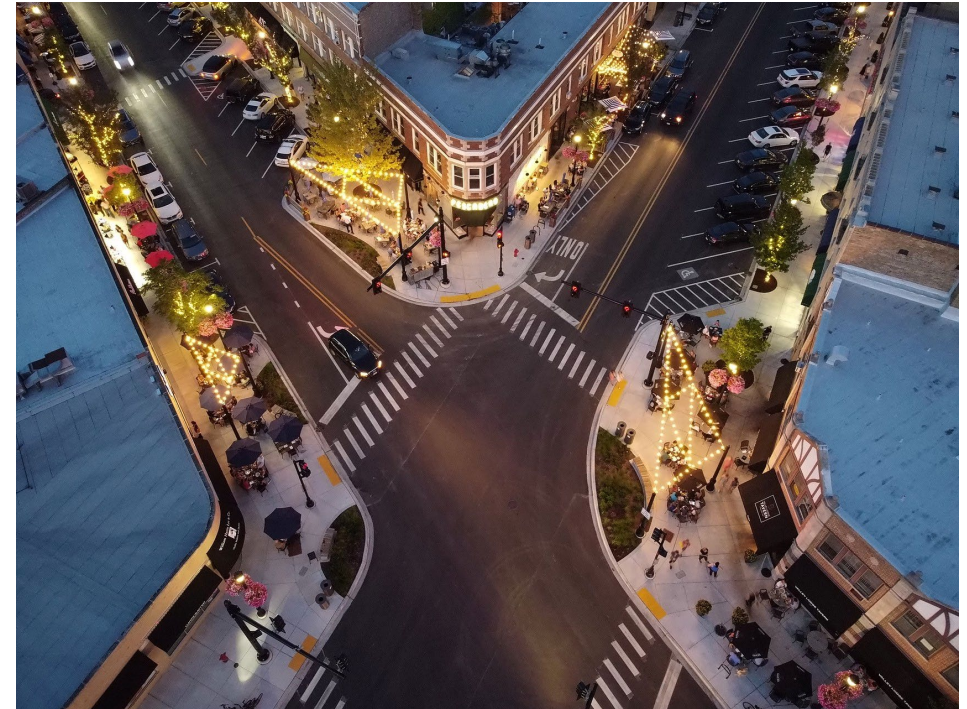
Example of improved traffic signals, lighting and traffic calming measures
