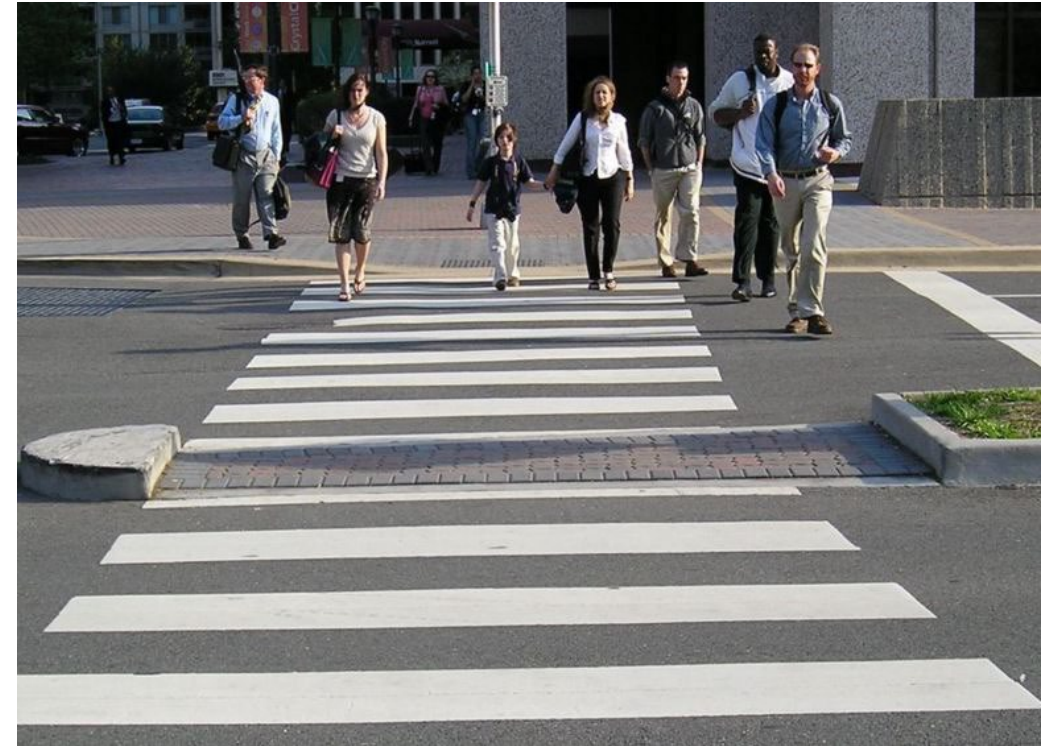
Example of enhanced crossing with median
